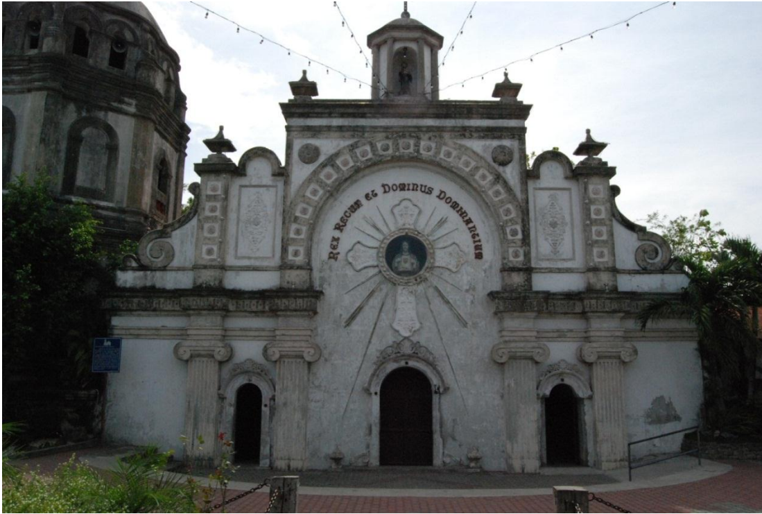
San Guillermo Façade. The entrance was originally a second floor window.
